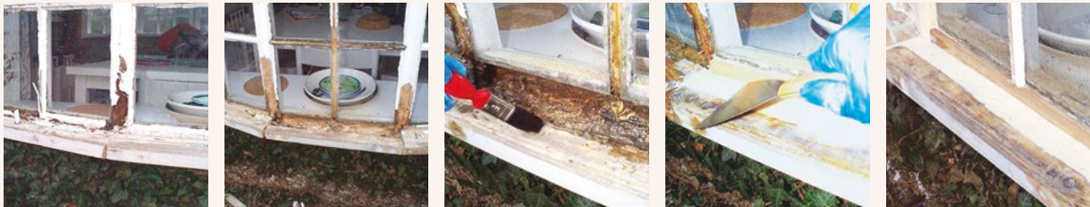
WINDOWS - DOORS - FRAMES - SOFFITS - FASCIA BOARDS - WOODEN CONSTRUCTION COMPONENTS
